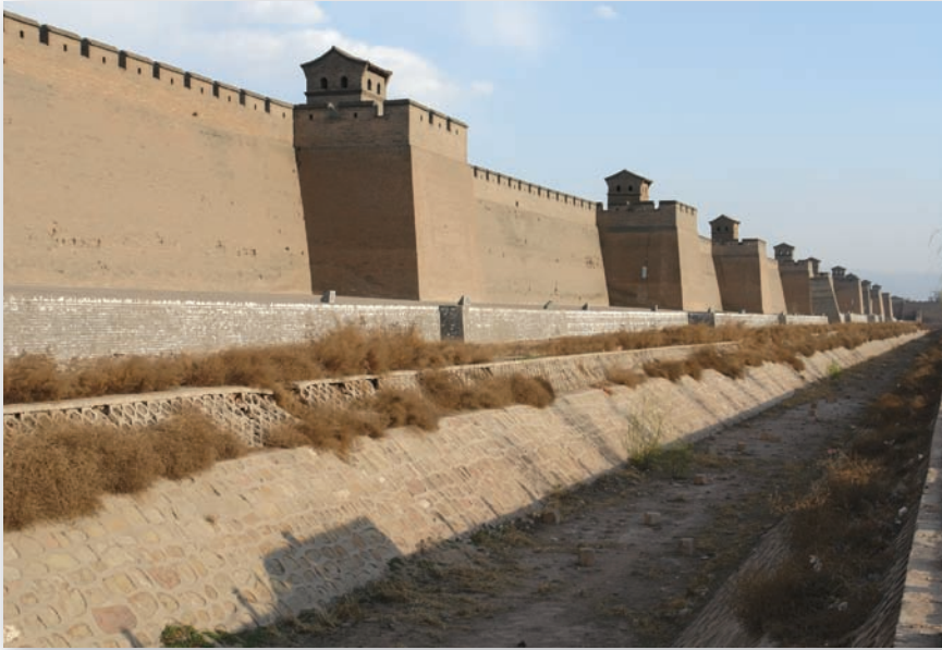
This is but one small section of the western wall of Pingyao, China's finest surviving fortified city. 'Horse-faced towers' with two-storey guardhouses above them protrude from the wall at regular intervals.
