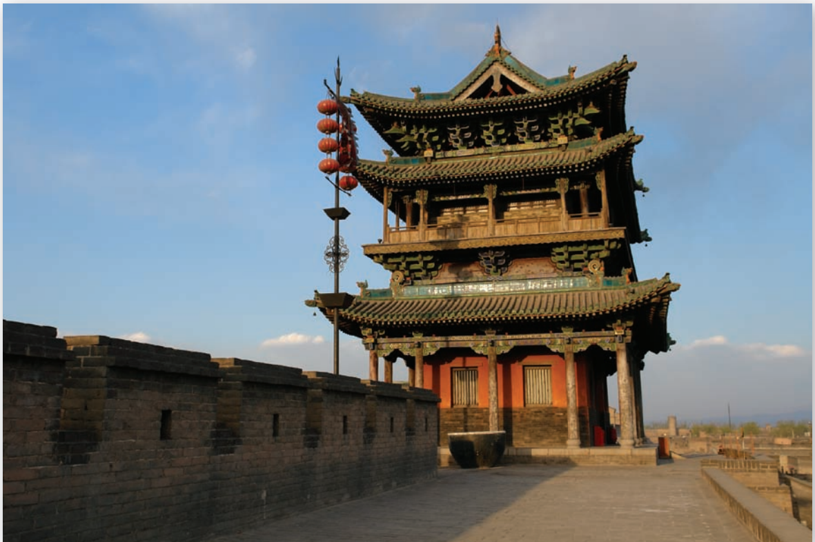
This beautifully restored wooden tower stands over the northern gateway of Pingyao.
