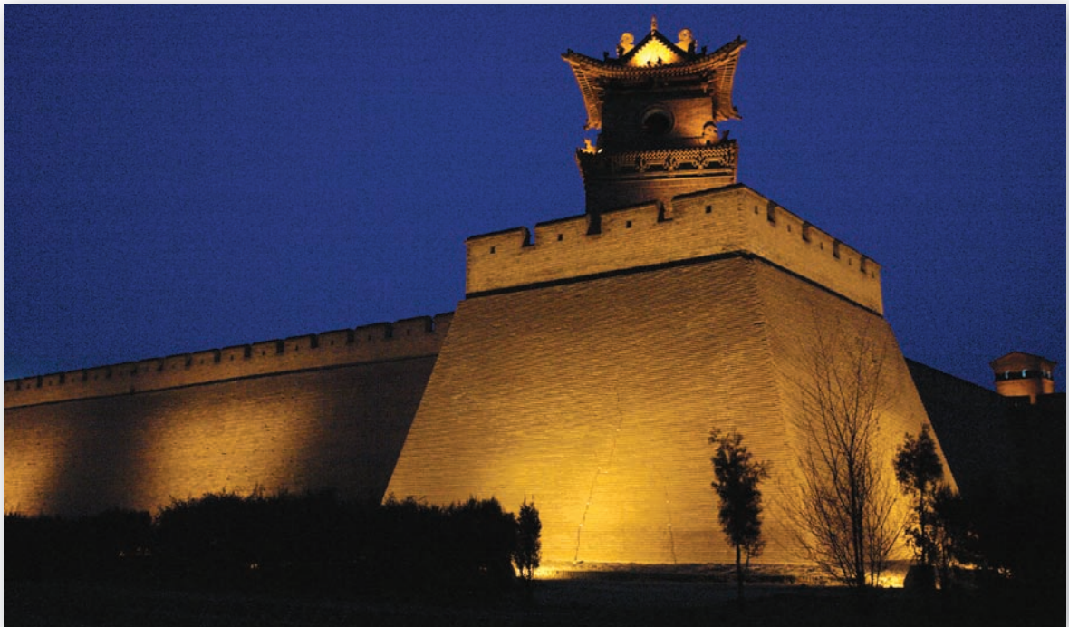
The tower at the corner intersection of the northern and western walls of Pingyao under floodlights.
