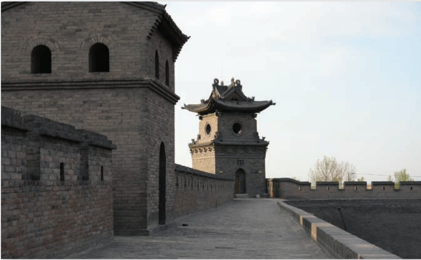
This delicate corner tower stands at the intersection of the northern and eastern walls of Pingyao.
