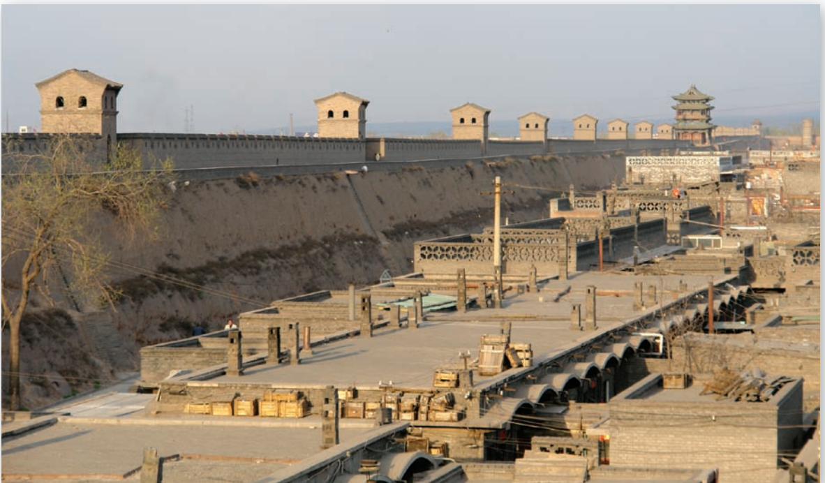
The northern wall of Pingyao as seen from a vantage point on the inside of the western wall. Its height is most impressive. Note the small parapet on the inner side and the pronounced slope. The northern gate tower stands out in the setting sun.
