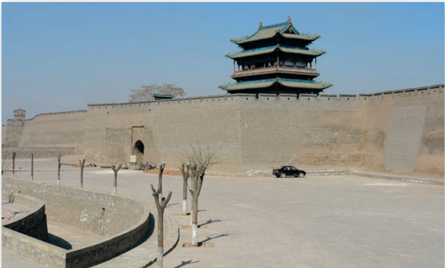
The area outside the southern gate of Pingyao is currently being landscaped, and the extent of the clearance brings out the imposing nature of the bare walls. The solitary motor car provides an indication of scale.
