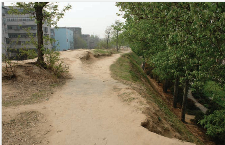
The Shang dynasty wall made from rammed earth at Zhengzhou. These are probably the most ancient surviving walls in China, and are used today almost as a public park.
