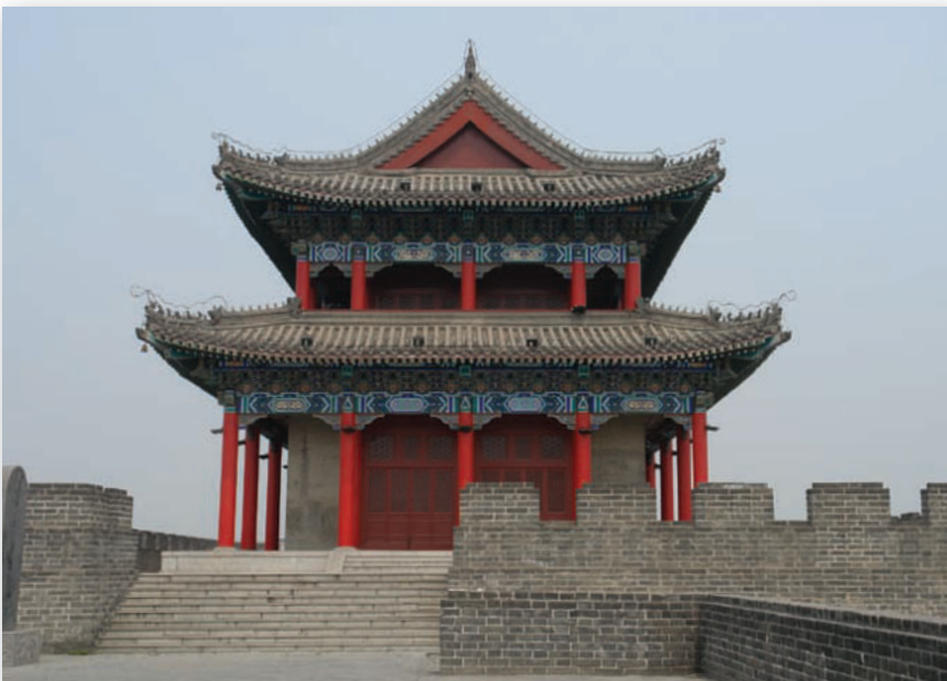
The two-storey pavilion on top of the western gate at Kaifeng. This is a typical construction found in many sites. Details of the brick nuqian (parapets) round the top of the wall may also be noted.
