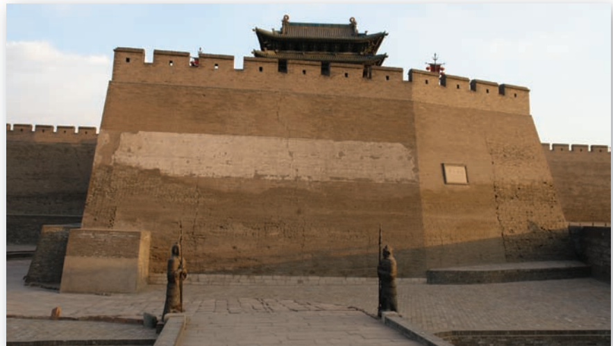
This view of the northern gateway of Pingyao illustrates the wengcheng principle whereby the gate is entered at 90 degrees from the passage through into the city.
